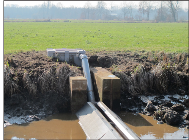
Figure 10: Picture of the crab trap in Grobbendonk, installed in 2018 by the Vlaamse Milieumaatschappij (Flemish Environmental Agency). Credits: Rotor vzw, Brussels, Belgium.
