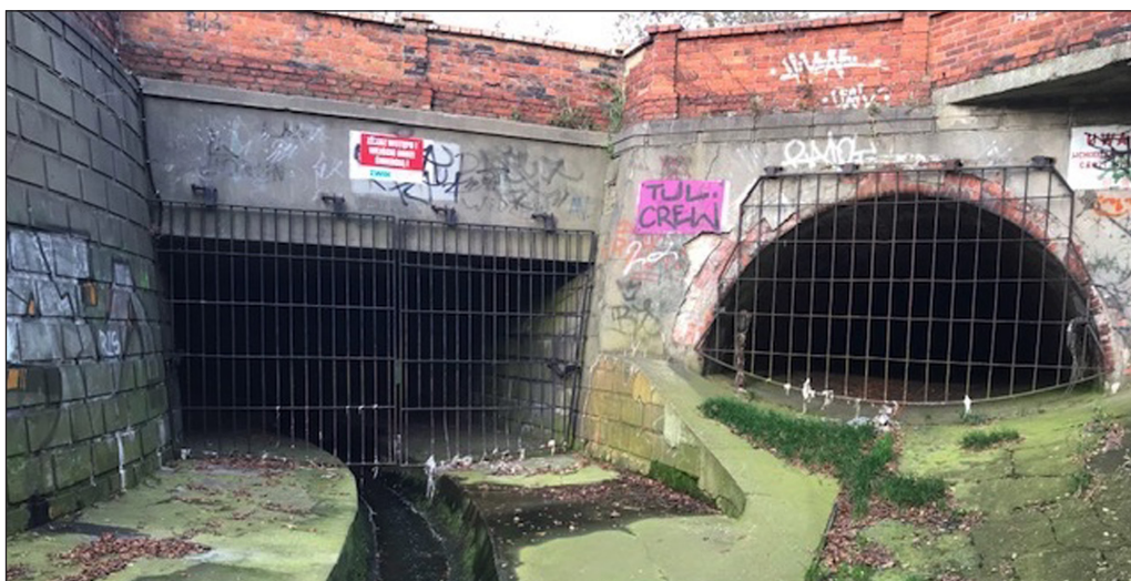
Figure 15: Gridded culverts on upriver end of Jasień River. (Photo by Philip Hayward, October 2022).
