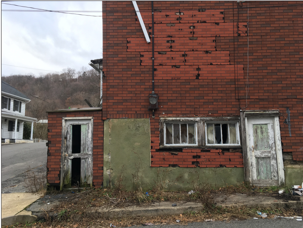
22. On a walk through an alley, I pause to notice the texture of a wall.
